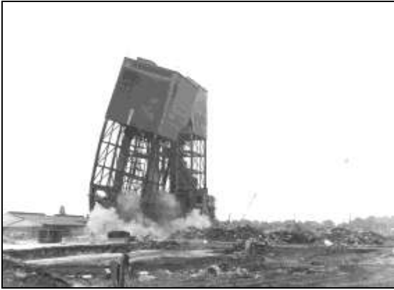
Warsop Main Colliery : Demolition of the First Headstock 23 rd October 1991 (Courtesy of Kevin Cantrell)
