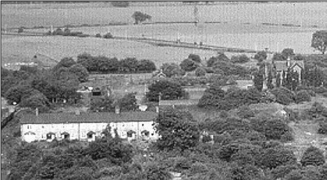
Above: Rhein O' Thorns (Mechanics' Cottages) and Rock House (Manager's House) (Taken from the headstocks by PC Cook in 1968)
