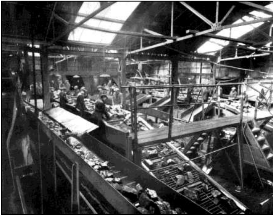
Above: Screening Coal at Warsop Main Colliery
