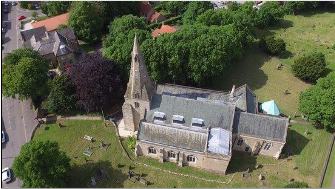
IMAGE 03 The Baroness took us to the church of St Mary & St Laurence. A mix of Saxon, Norman and Victorian architecture that has survived fires in 1897 and 1960 as well as having to be underpinned in the 1990s due to mining subsidence.
